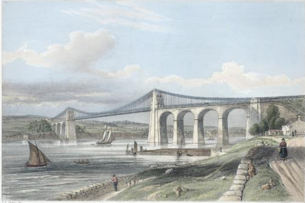
THE SUSPENSION BRIDGE OVER THE MENAI. Length of each tower 60 feet; height of tower from the top of the pier to the top of the chain 100 feet; height of the chain from the top of the pier to the top of the tower 100 feet; height of the tower from the top of the pier to the top of the chain 100 feet; height of the tower from the top of the pier to the top of the chain 100 feet.
